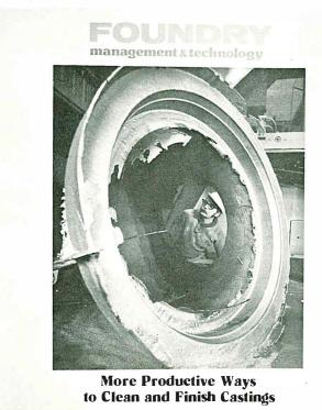
A Wheelabrator 96-inch Swing Table leads off the cover story — "More Productive Ways to Clean Castings" — in the current issue of Foundry Management and Technology. Pictured is the inspection of a large pipe elbow casting immediately after blast cleaning in our Swing Table. No-bake sand is broken up and reclaimed in the casting cleaning operation at the Backman Foundry, Provo, Utah.
